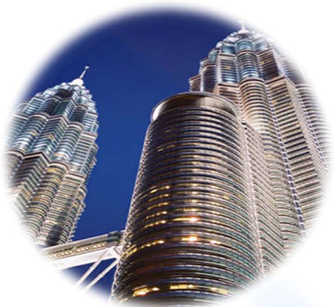
Protecting HVAC System Investment
